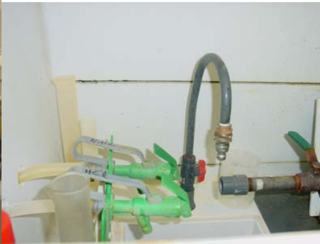
After: GoatThroat delivers technical grade HCl and Nitric Acid, plumbed in through side of fume hood, dispensed with remote tap. Acid cost reduced to $.20 per unit.
