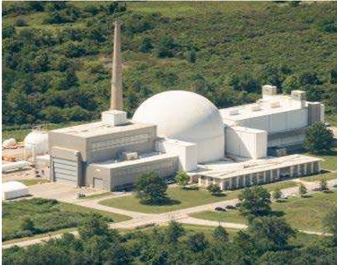
Figure 9: Space Environments Complex (SEC) aerial view.
